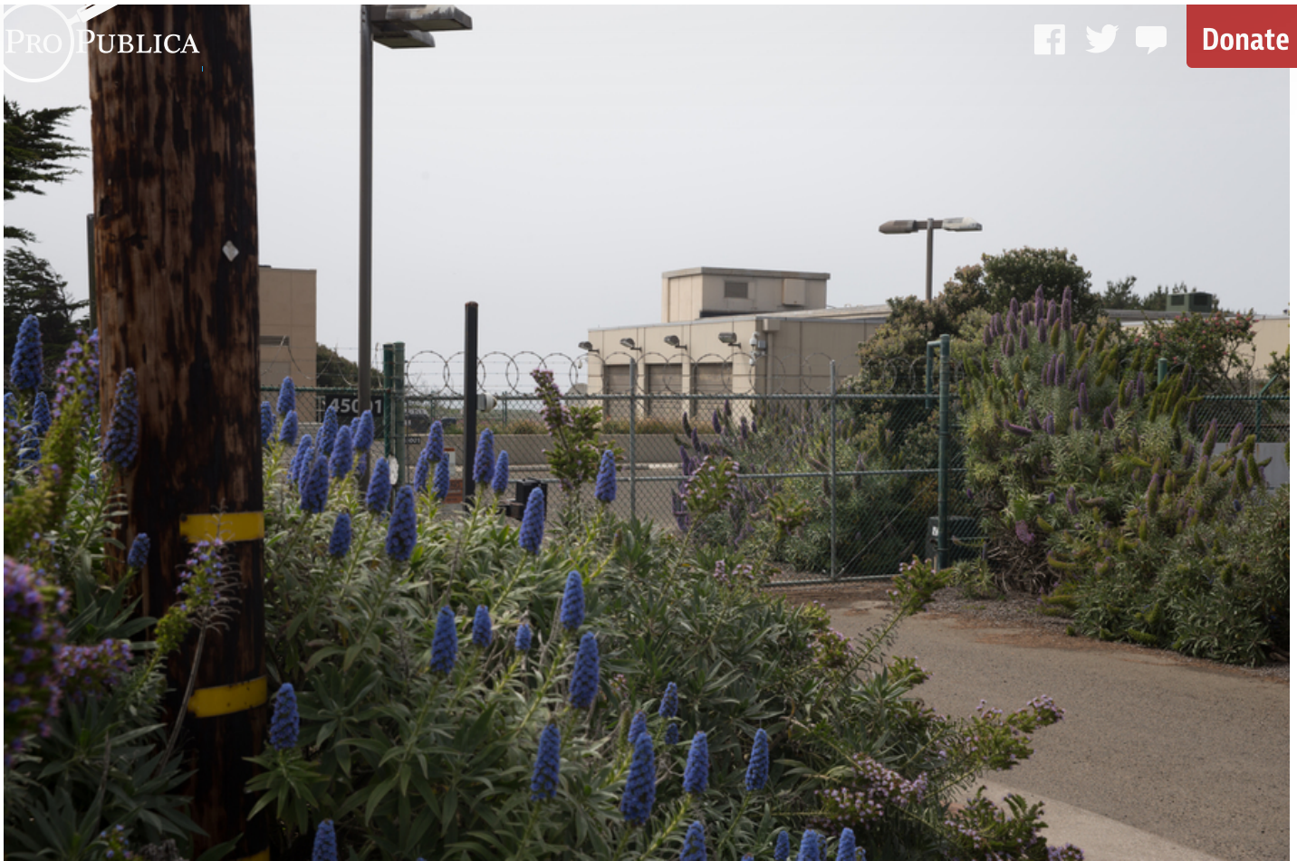
AT&T's cable station in Point Arena, California. NSA collection at this site was temporarily disrupted after the 2011 Japanese earthquake damaged the undersea cable. (Henrik Moltke for ProPublica)
